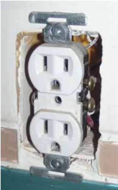
Receptacle is "back-wired"
